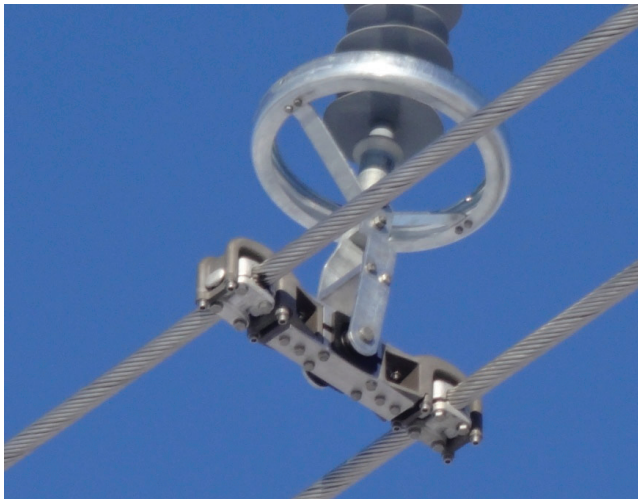
The spacer attaches to the conductor on both ends.
