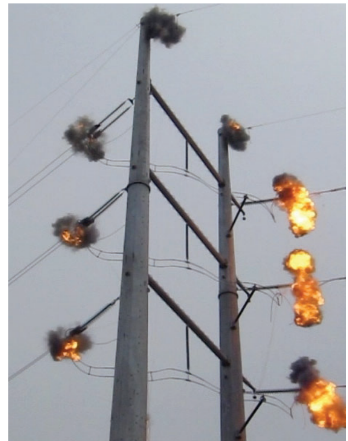
Use of implosive connection devices
